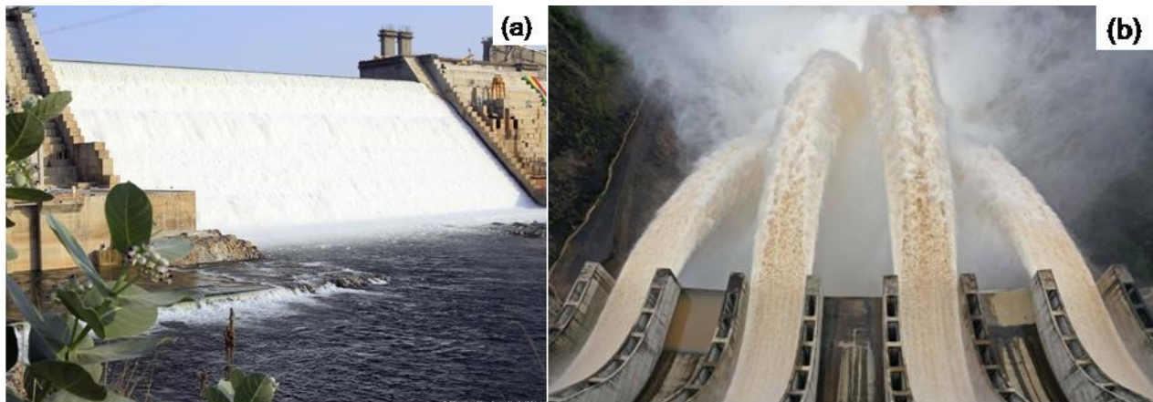
Figure 1. Aerated flows in hydraulic structures: (a) flow over the emergency spillway of the Grand Ethiopian Renaissance Dam; and (b) water jets from the spillway of the Gibe III Dam, Ethiopia (Photographs courtesy of Studio Pietrangeli Consulting Engineers, Italy).
